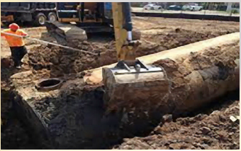
Underground Storage Tank (UST) Removal
