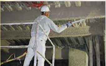
Spray-Applied Fireproofing
